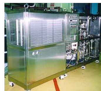
Contactors in use at Wolsung NPP
