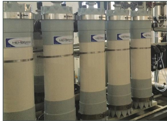
Liqui-Flux® W10-07 Ultrafiltration Modules as pre-treatment to reverse osmosis
